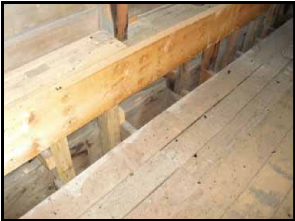
47. SUPPORT OF ATTIC FLOOR JOISTS AT EATS GABLE END WALL.
