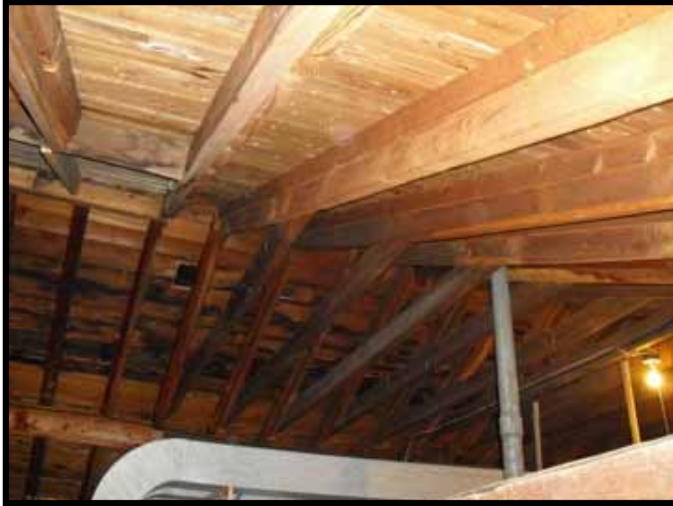
53. ROOF RAFTERS HAVE SECOND 2X MEMBER SISTERED ON ONE SIDE. PERHAPS TO STRAIGHTEN THE ROOF DECK BOARDS.
