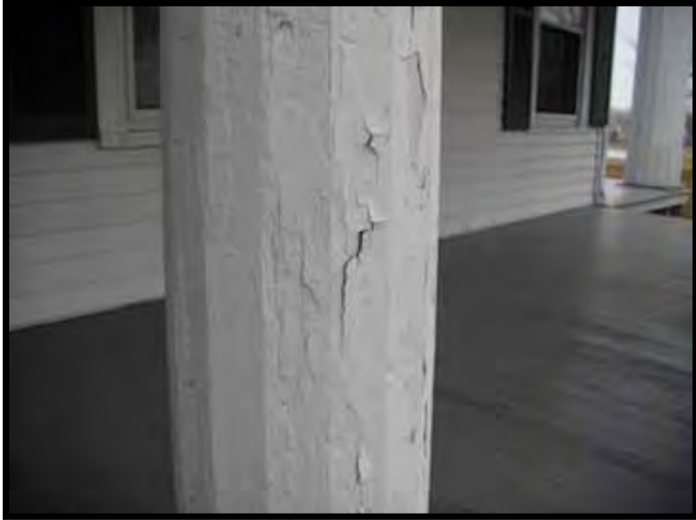
63. SOUTH PORCH COLUMN.
