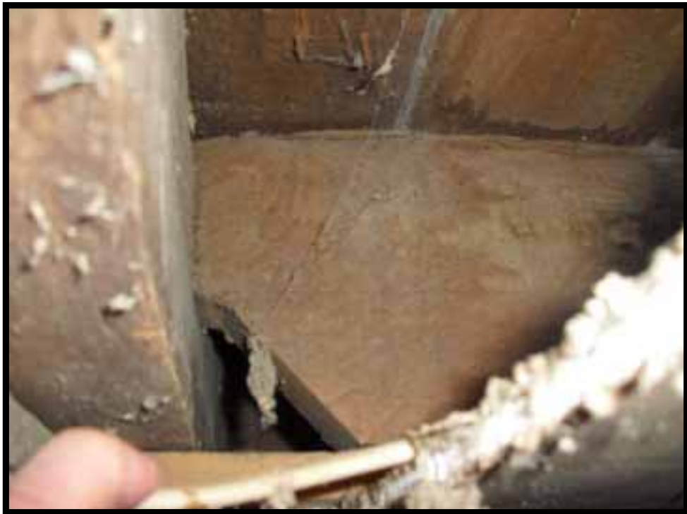
12. JOISTS ABOVE S-W CORNER BASEMENT ROOM MORTISE INTO CENTRAL BEAM.
