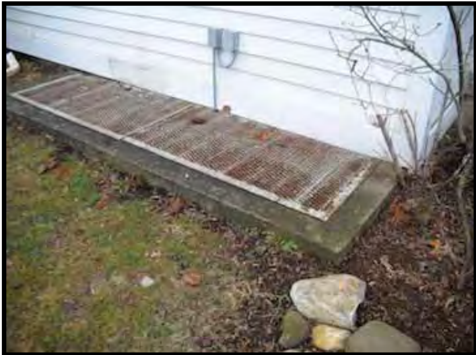
70. SOUTH WEST CORNER OF NORTH WEST WING.
