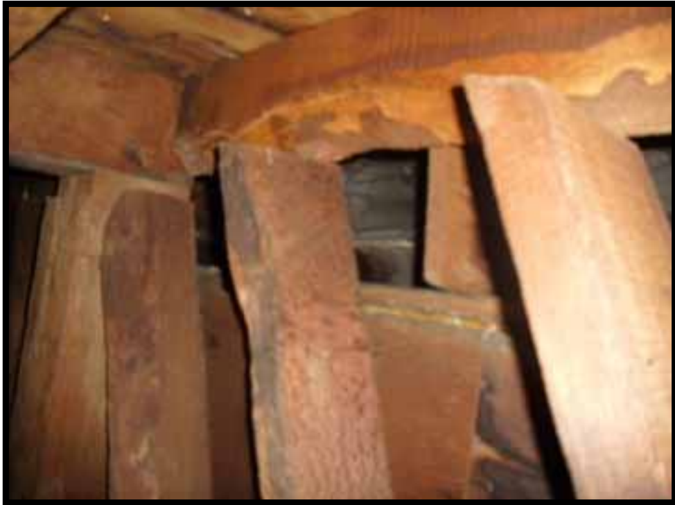
45. CLOSE UP OF GABLE END WALL FRAMING AT ROOF.
