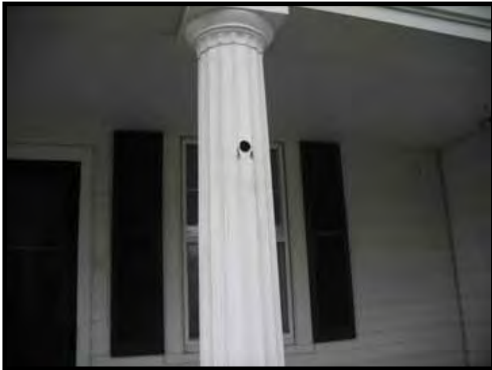
56. TOP OF NORTH PORCH COLUMN.
