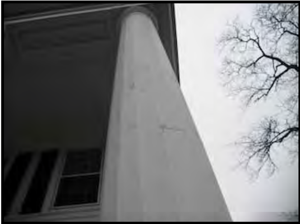
58. NORTH EAST CORNER COLUMN.
