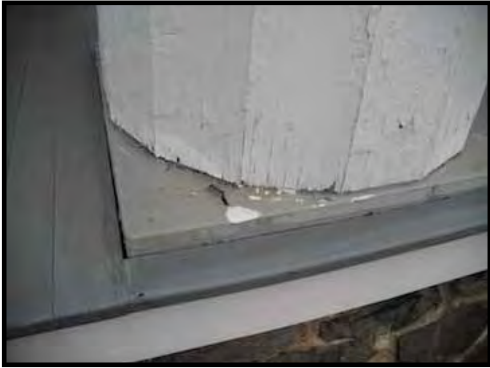
59. BASE OF EAST PORCH COLUMN.
