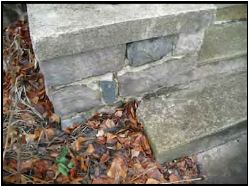
64. STONE FLANKING EAST EXTERIOR STAIRS.
