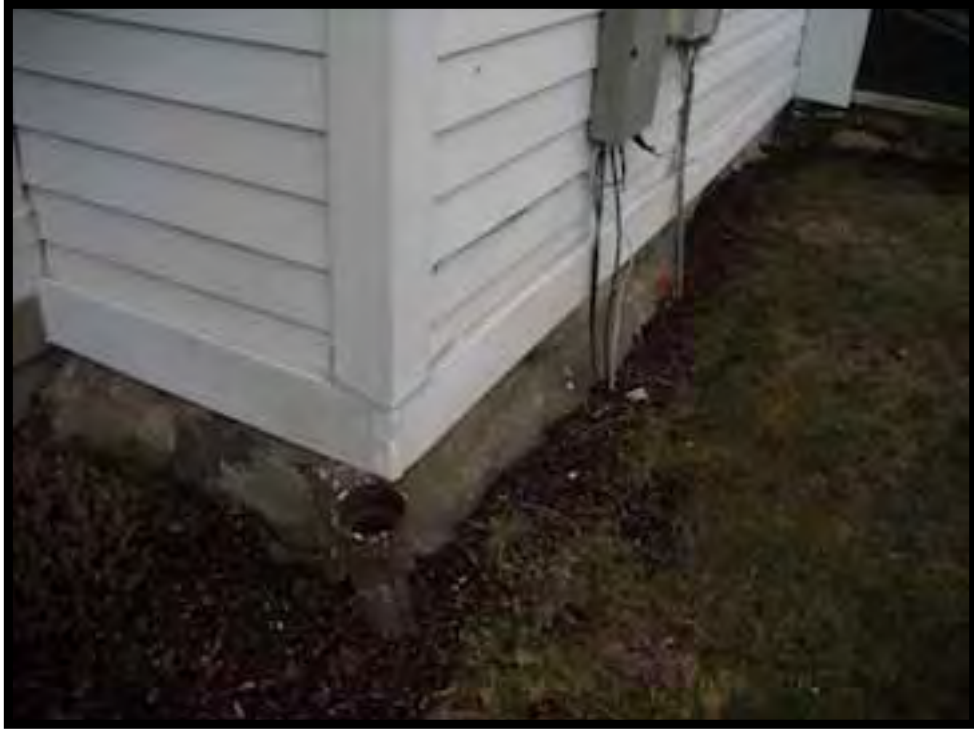
69. FOUNDATION AT NORTH WEST CORNER OF SOUTH WEST WING.
