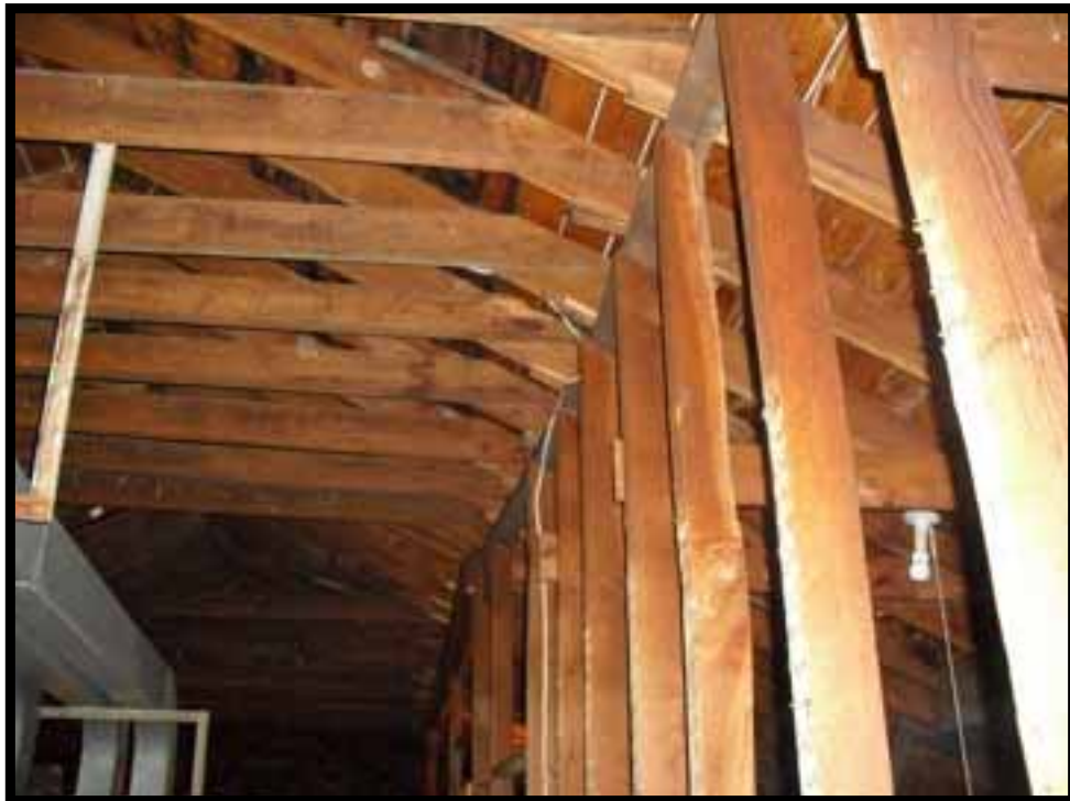
24. ROOF FRAMING LOOKING EAST.
