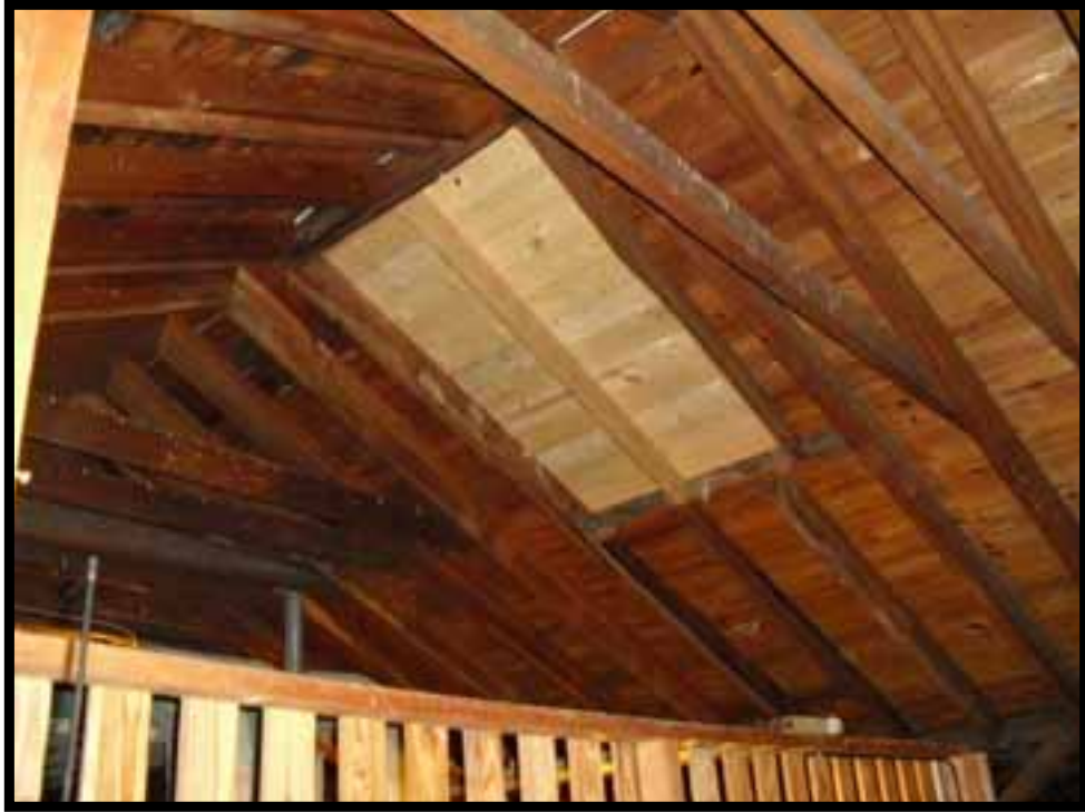
31. MOST RAFTERS HAVE COLLAR TIES EXCEPT AT AREA OF FORMER SKYLIGHT.
