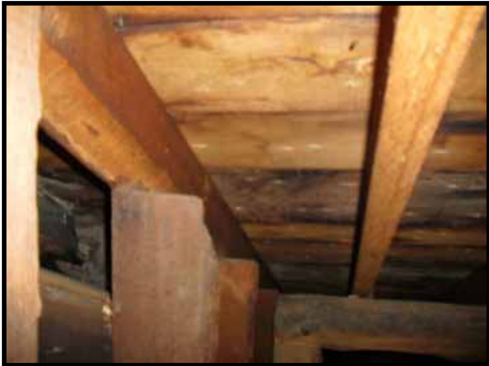
46. CLOSE UP OF GABLE END WALL FRAMING AT ROOF.
