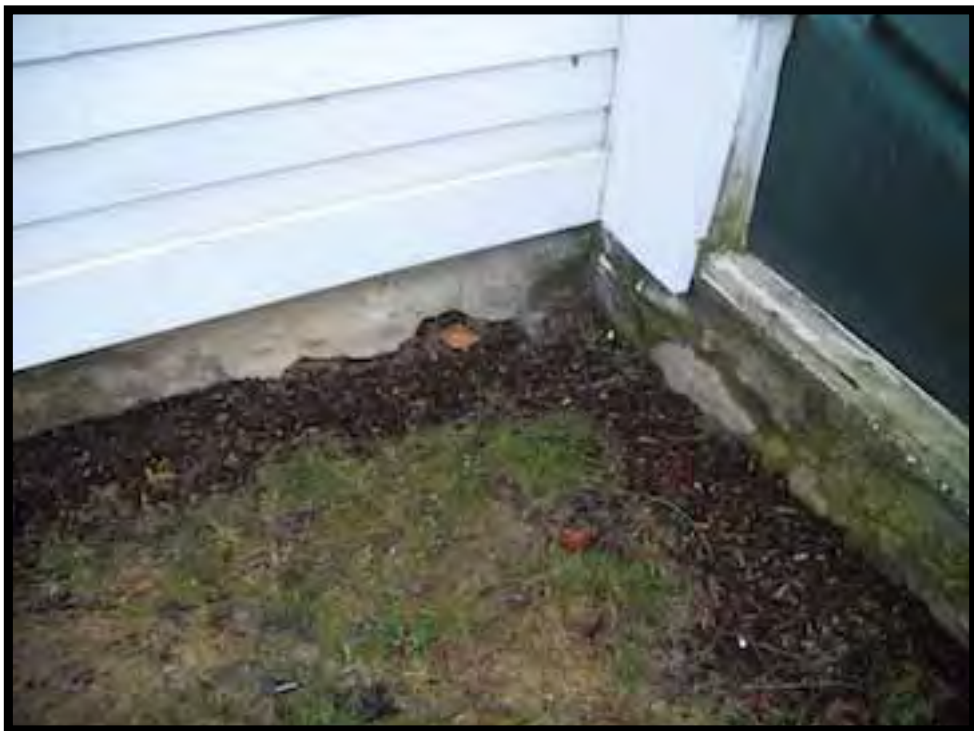
68. FOUNDATION ADJACENT TO CELLAR DOOR.
