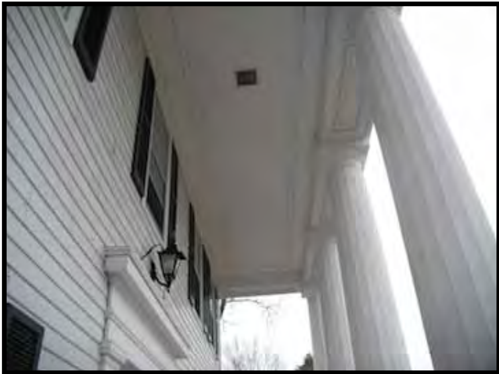
60. EAST PORCH LOOKING NORTH AND UP.
