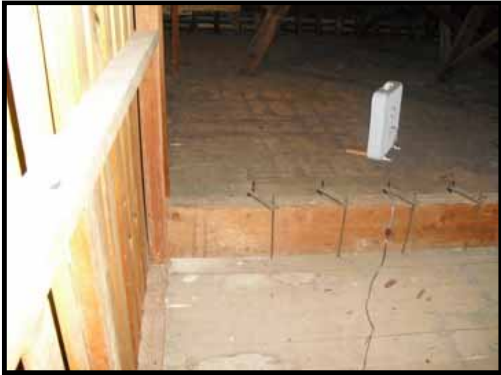
27. NON ORIGINAL BEAM HANGING ATTIC FLOOR STRUCTURE.
