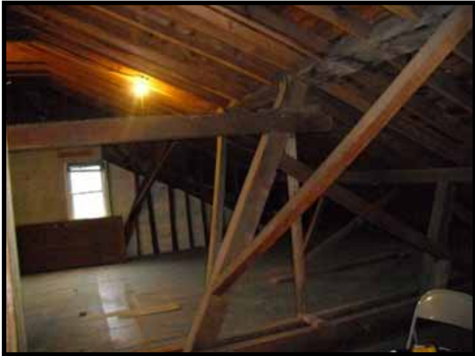
35. LOOKING NORTH WEST AT ROOF FRAMING IN NORTH WEST CORNER ATTIC.
