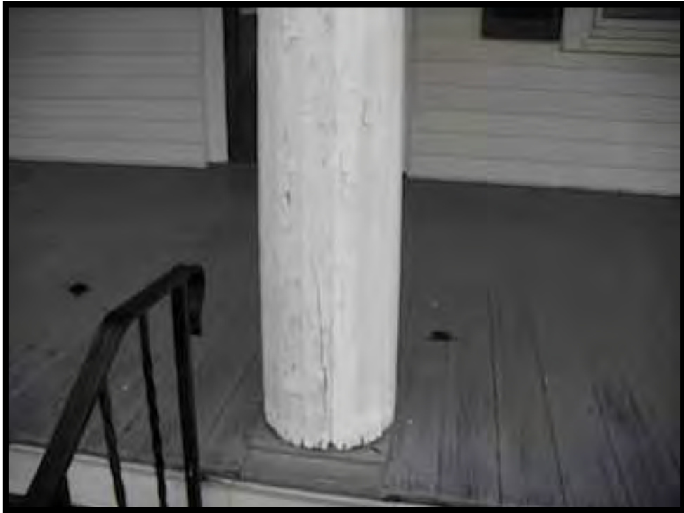
61. SOUTH PORCH COLUMN.
