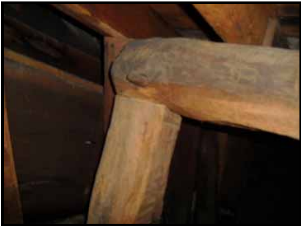
44. PEGGED MORTISE AND TENON JOINERY OF ROOF PURLINS AND COLUMNS.
