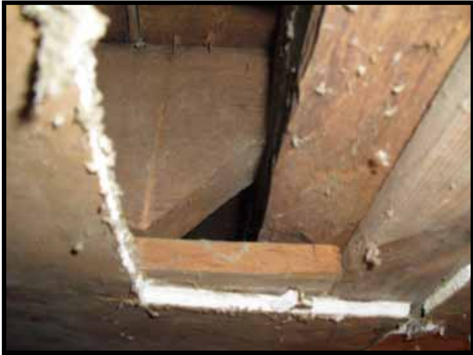
11. JOISTS ABOVE S-W CORNER BASEMENT ROOM MORTISE INTO CENTRAL BEAM.
