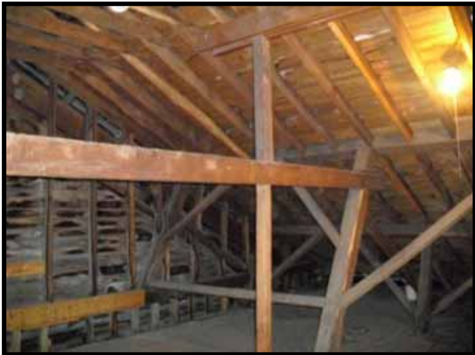
42. FRAMING IN SOUTH EAST CORNER OF ATTIC.
