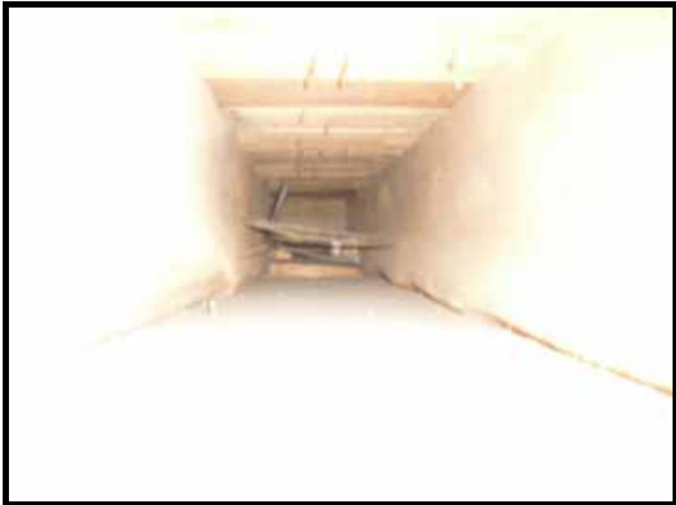
4. SPACE BETWEEN 3X10 FIRST FLOOR JOISTS.
