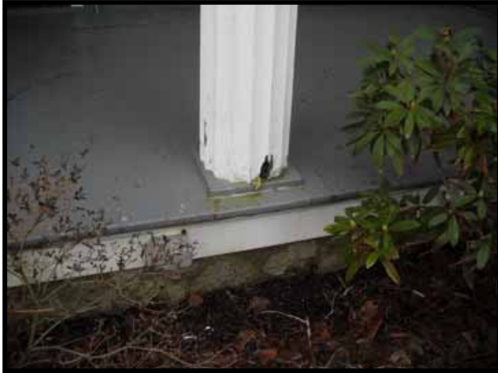
55. BASE OF NORTH PORCH COLUMN.
