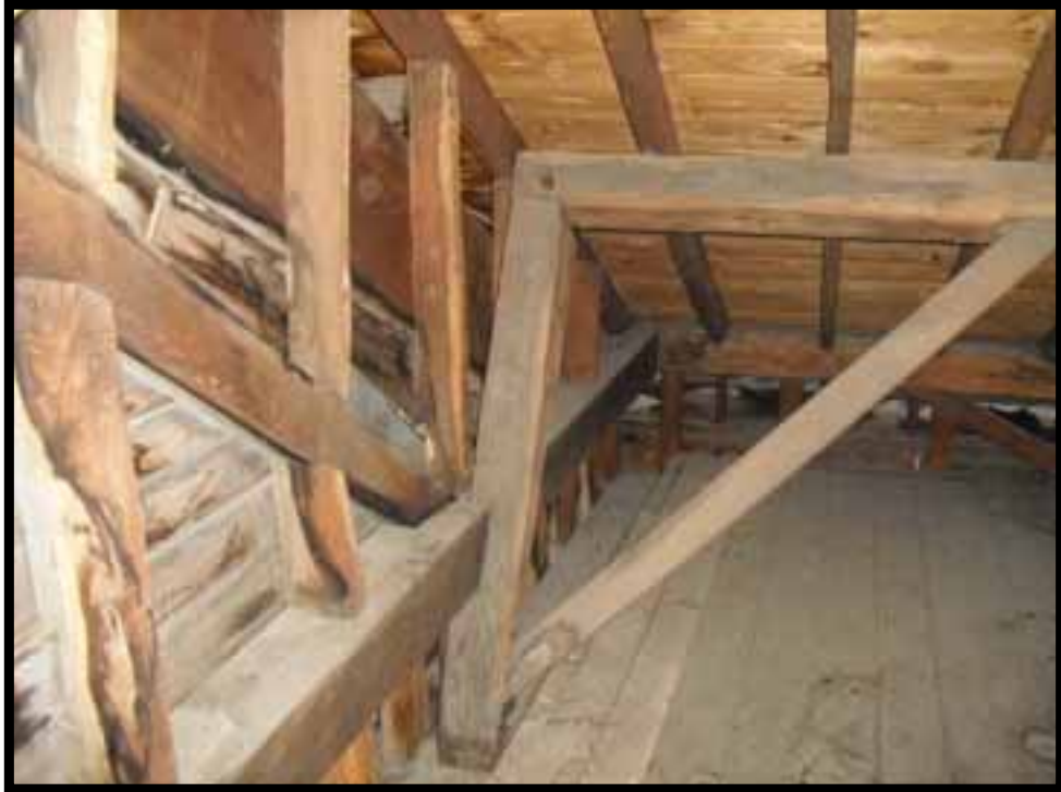
37. DETAIL OF ROOF AND GABLE WALL FRAMING.
