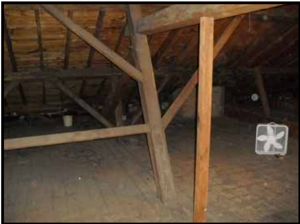
50. ATTIC FLOOR AND ROOF FRAMING LOOKING NORTH.
