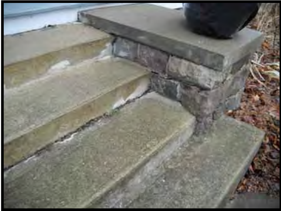
65. STONE WALL FLANKING EAST EXTERIOR STAIRS.
