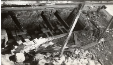
Steel beams support the house
